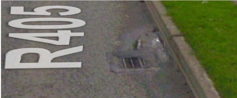
stretch nearest to Celbridge (between the Liffey bridge and Hazelwood estate) has no cycle lanes. The road space that cyclists share with vehicles has many poorly designed drains with notable dips which result in cyclists swerving around them.
